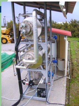
Figure: View of the evaporator (installed on site)
